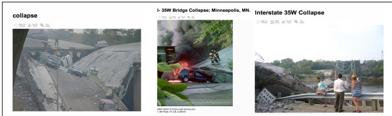
Figure 7: Images Taken Immediately After the Minneapolis Bridge Collapse
